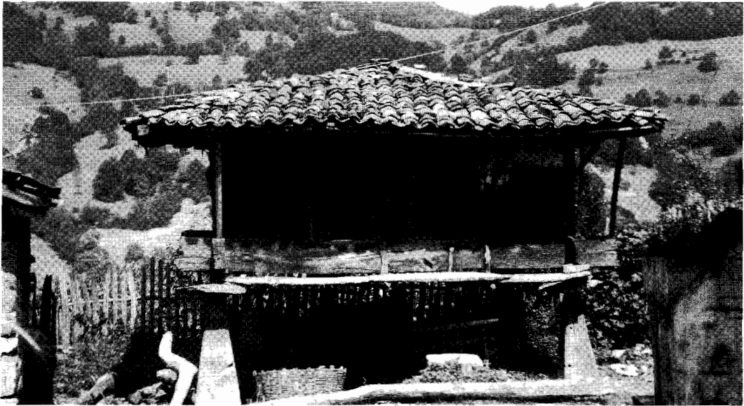
Fig. 2. Elevated granary, Asturias, Spain. Square plan, posts with rat-guards, wooden walls, no ventilating devices. Photo: F. Sigaut 1979.
